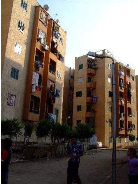
Figure 4, Ezbet-Haridy after rehabilitation project. (Abouelmagd,S. , 2012)
