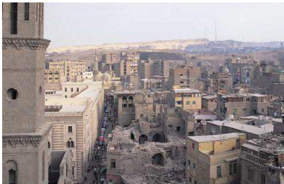
[fig. 7] Eldarb El-Ahmar, deteriorating area. Source (AGTC, 2001)
