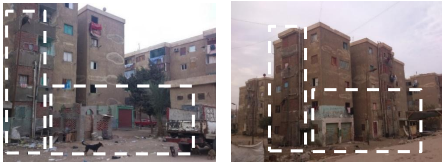
Figures 11 and 12, show different examples for the physical changes in Nahda city, this includes the transformation of the ground floors to commercial shops and the closing of balconies (Photos taken by the authors, June 2013)
