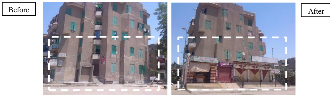
Figures 9 and 10, show the physical changes in one of Suzan Mubarak building (right), compared to another building on the project without transformation (left) (Photos taken by the authors, August 2014)
